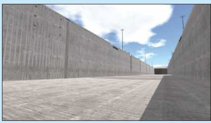
WHOLE LOTTA CONCRETE: Chamber wall monoliths line an engineering representation of the future New Lock at the Soo, in Sault Ste. Marie. A $213.8 million contract for the work was awarded to Kokosing Alberici Traylor last month.
