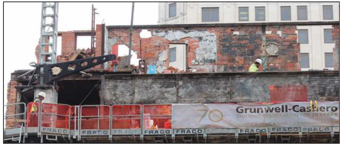
DISMANTLING THE FACADE of the National Theater in Detroit are Anthony LaFata and Ryan Harding of Bricklayers and Allied Craftworkers Local 2. Facade elements will be rehabilitated, stored and then re-built on site. The masons are employed by Grunwell-Cashero.
