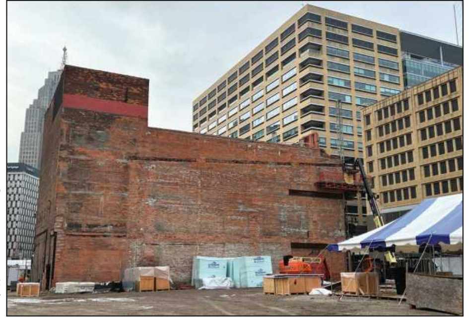
DISMANTLING THE FACADE of the National Theater in Detroit are Anthony LaFata and Ryan Harding of Bricklayers and Allied Craftworkers Local 2. Facade elements will be rehabilitated, stored and then re-built on site. The masons are employed by Grunwell-Cashero.
